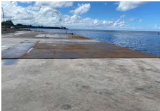
CARICOM Wharf Quay Phase II
