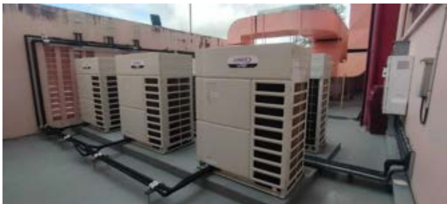
Replacement of HVAC System and Associated Works at the UWI Sports and Physical Education Centre
