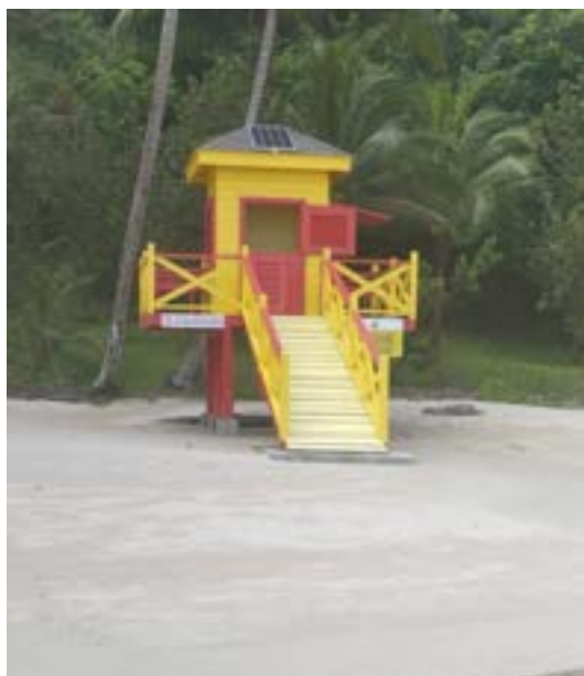
Upgraded Lifeguard Tower at the Las Cuevas Beach Facility
