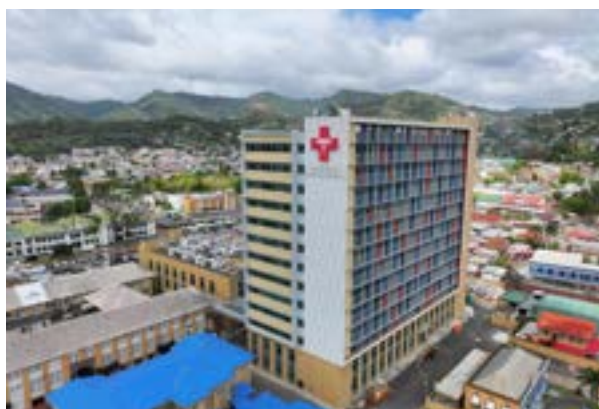
External Eastern Side of the Central Block, Port of Spain General Hospital
