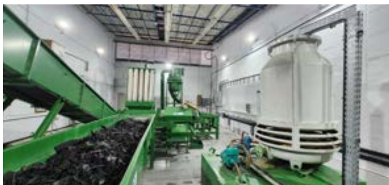
Rubber Crumb Facility, San Fernando Technical Institute
