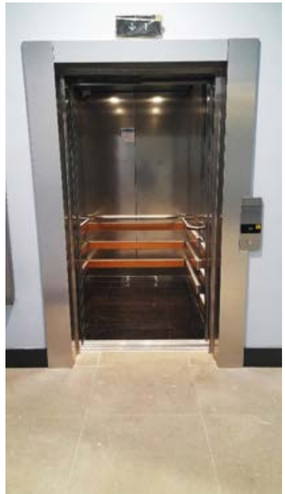
Lift at the New Terminal of the ANRRIA
