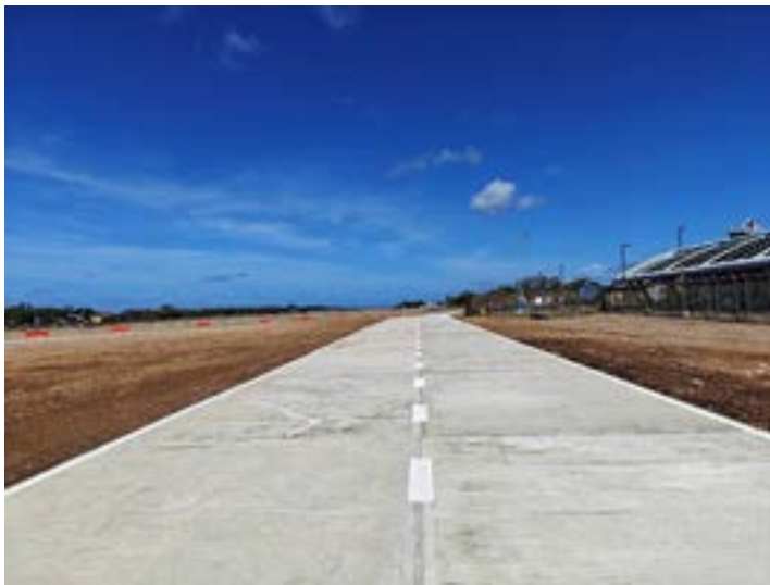
Perimeter road at the New Terminal of the ANRRIA
